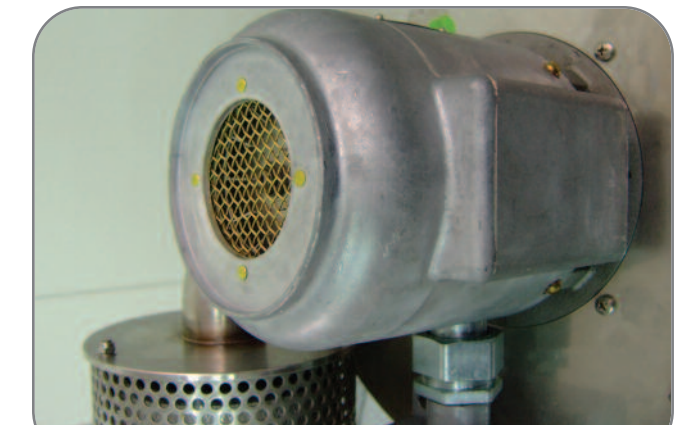
Explosion-proof, totally enclosed fan cooled (TEFC) motor
